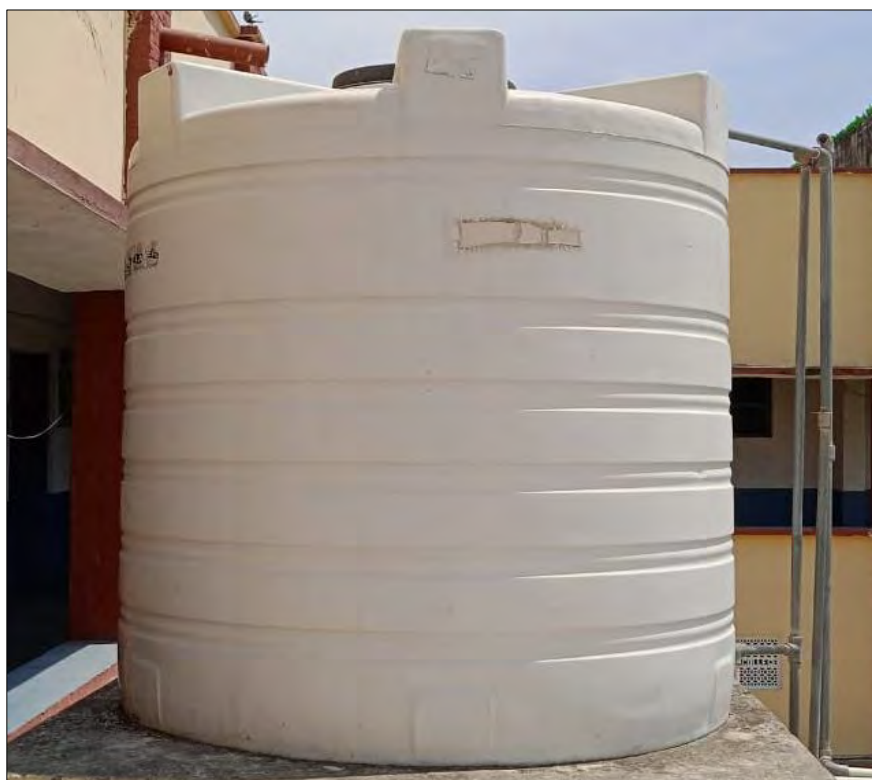
Fig 2.3 Water storage tank in college
